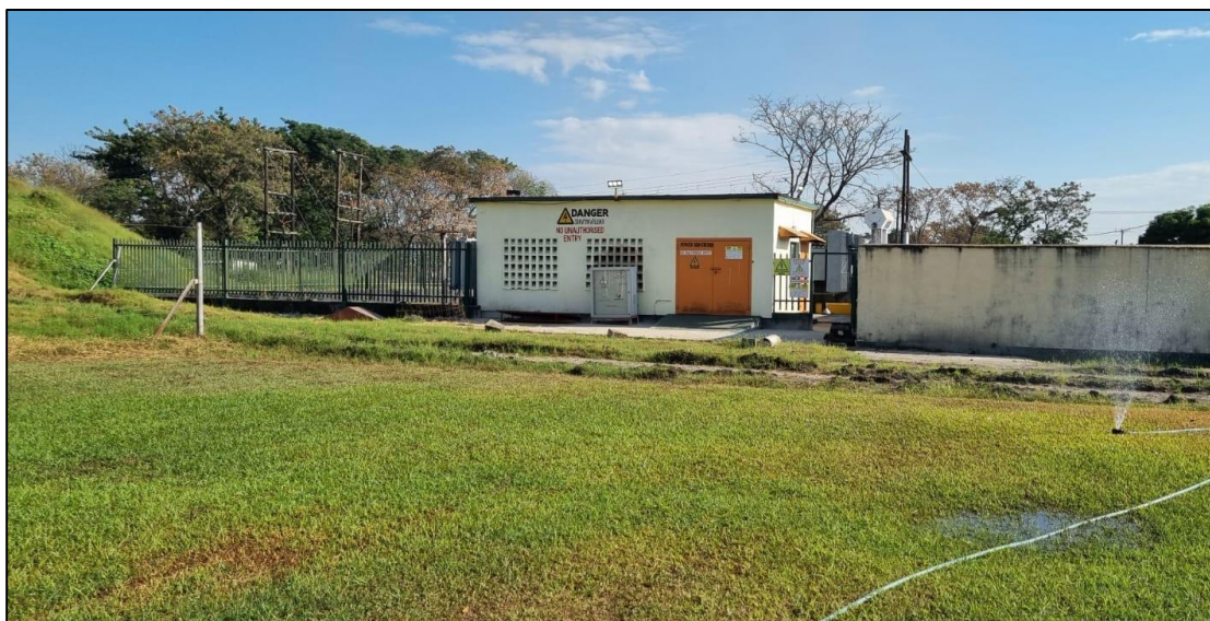
FIGURE 2.5: AREA PROPOSED FOR THE LAYDOWN OF CONSTRUCTION MATERIAL
