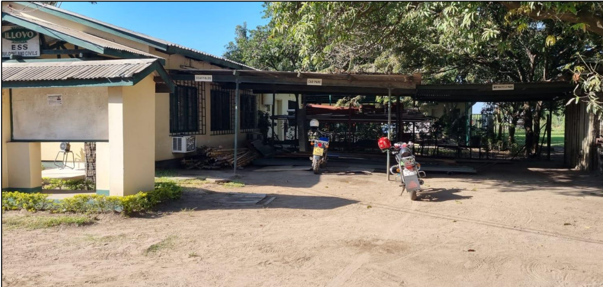
FIGURE 2.2: EXISTING FACILITIES TO BE UTILISED FOR ACCOMMODATION OF SEMI-SKILLED LABOUR
