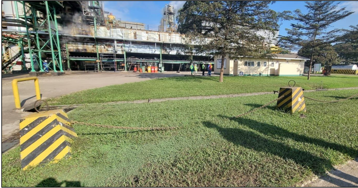
FIGURE 1.3: AREA WHERE NEW SHREDDER MOTOR AND NEW CRANE PREPARATION MCC BUILDING ARE PROPOSED
