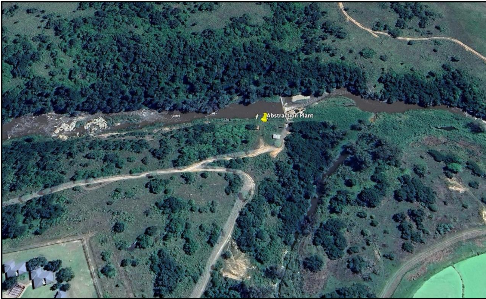
FIGURE 3: EMANZANA WATER TREATMENT WORKS UPGRADE ABSTRACTION POINT SEEKOEISPRUIT RIVER, EMANZANA (BADPLAAS), CHIEF ALBERT LUTHULI LOCAL MUNICIPALITY
