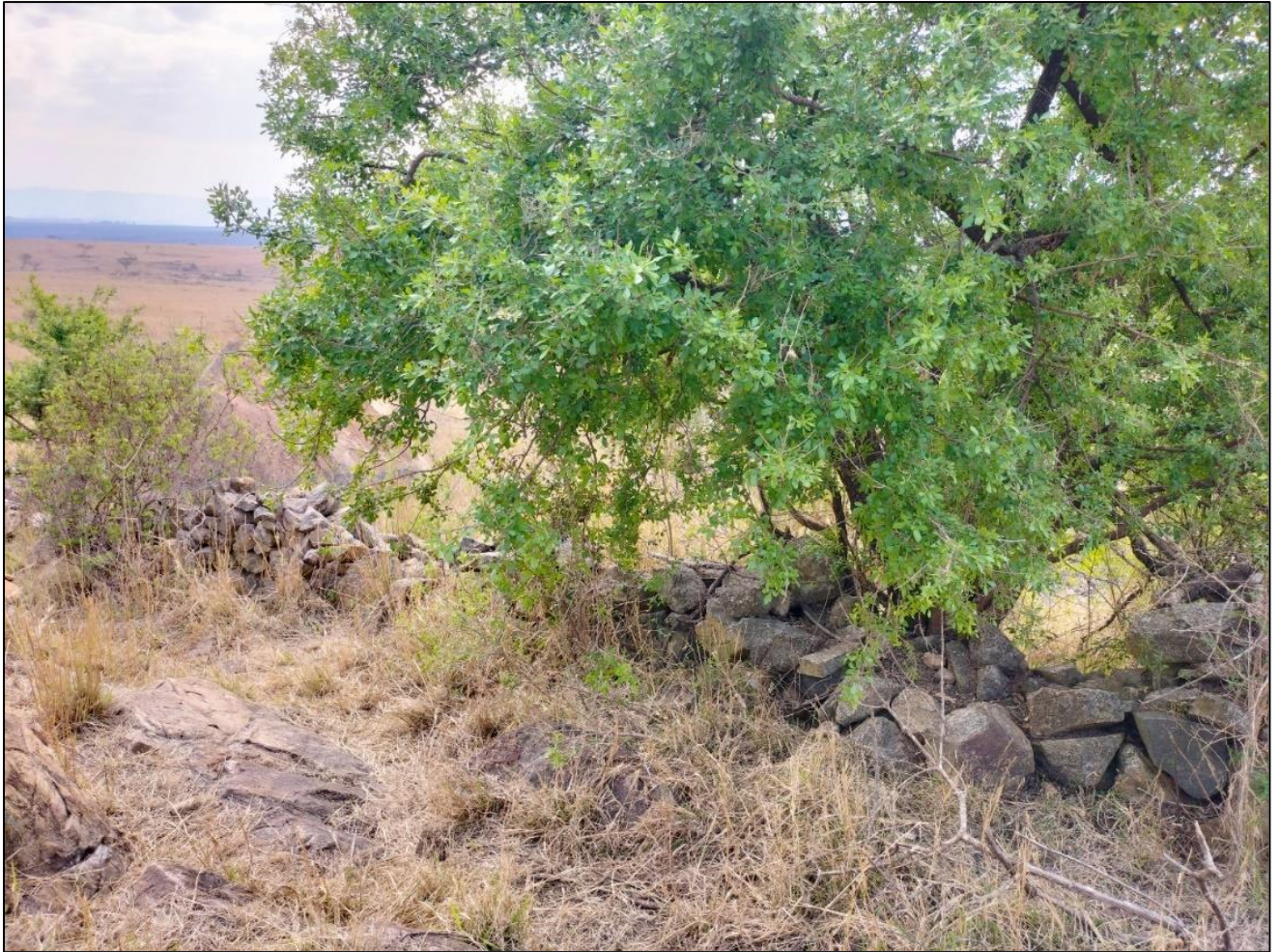
FIGURE 16: THE PROMINENT STONE WALL AT THE POD 9 SITE.
